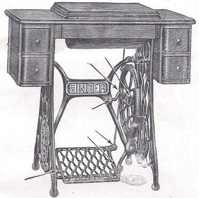
FIG. 11. OILING POINTS IN STAND
